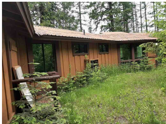
Walden building, rear
