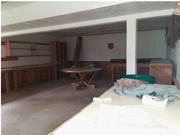
Interior, lower level
